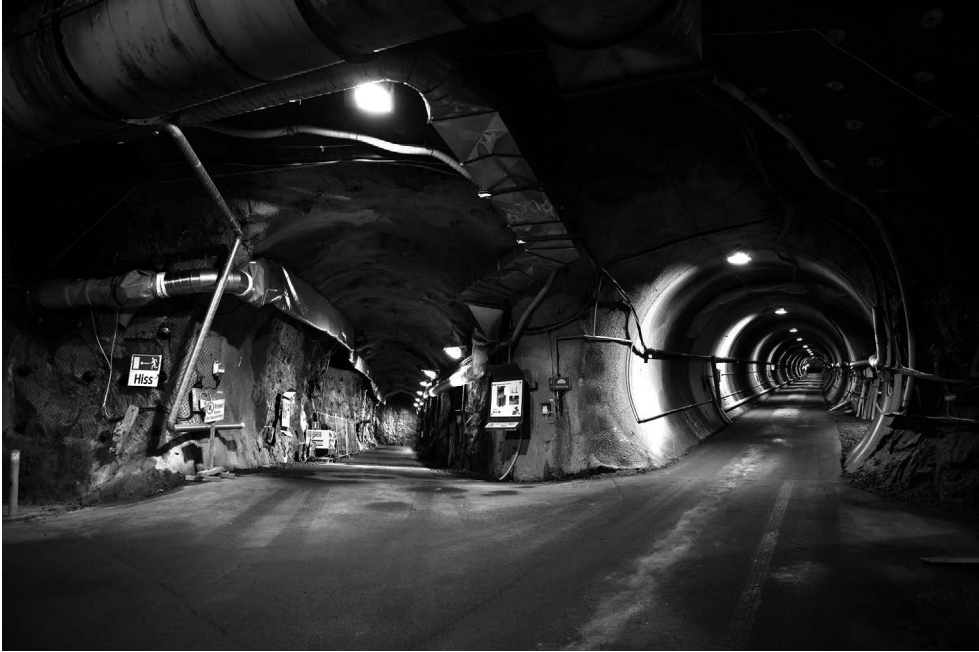
FIGURE 2.1 Inside the SFR at Forsmark, Sweden
